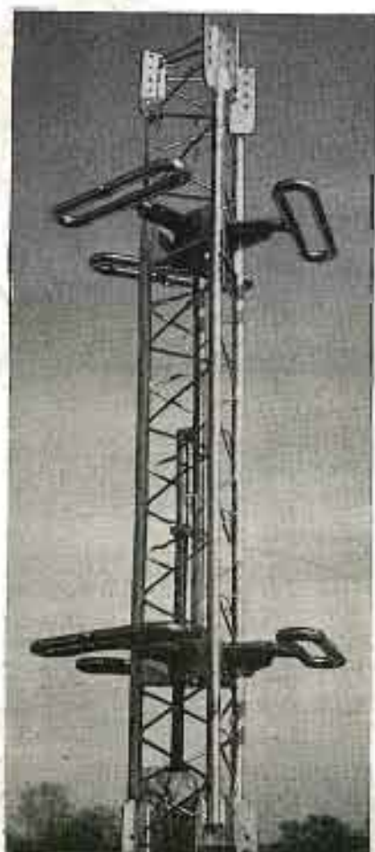
Figure 1 Pair of experimental triangular high band (channels 7 to 13) TV loops mounted on steel lattice structure,* which is 14" on side and built in 10' sections.
