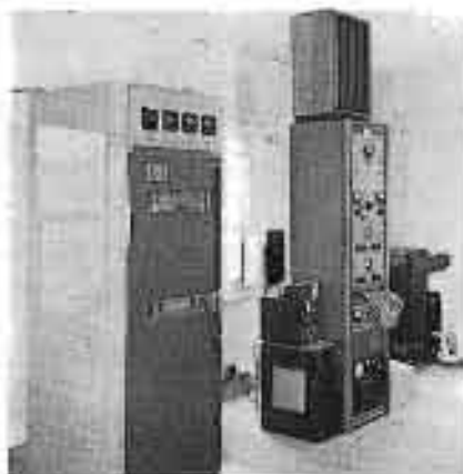
Interior view of equipment room at WTAL and WTAL-FM, Tallahassee, Florida. The AM transmitter at this station is a 5-kw job and the FM a 710-watt affair. A six-bay cloverleaf antenna is used with the FM transmitter. (Courtesy Caterpillar Tractor Company)
