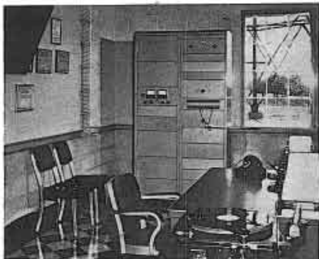
View of the main operating console, auxiliary turntable and other equipment at WSJS-FM. The bottom of the antenna may be seen through the window.
