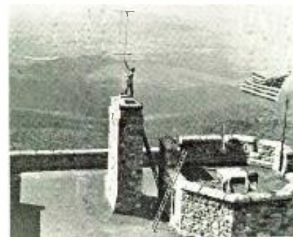
Tv receiving antenna atop the Castle at the summit of Whiteface Mountain in New York State being used to pick up signals from WRGB at Schenectady, 120 airline miles away. (Courtesy General Electric.)
