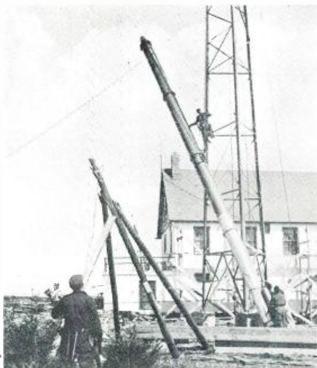
Erection of the first pylon antenna at the De Ruyter station.
