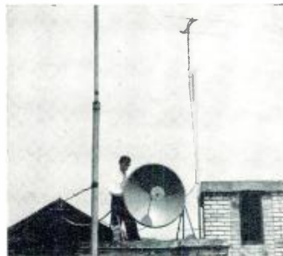
Microwave dishpan antenna atop the Ithaca Savings Bank Building which is used to beam programs to Connecticut Hill where they are channeled to the six stations in the network chain.
