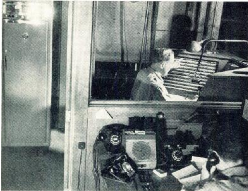
Relaying telephone calls to radio police cars patrolling the streets of Philadelphia. Cabinet at left houses remote control relay system for duplex operation.
