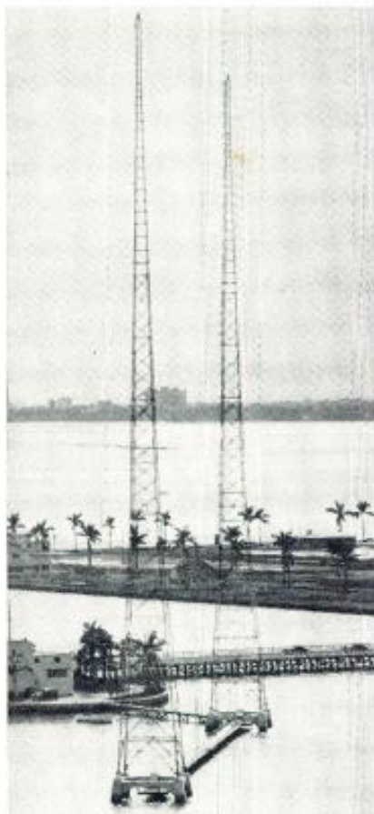
The 5 kw a-m island location of WQID, Miami, Florida. This type of installation provides excellent ground conductivity.
