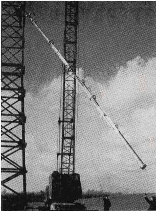
(Left) Erecting the circular antenna.
