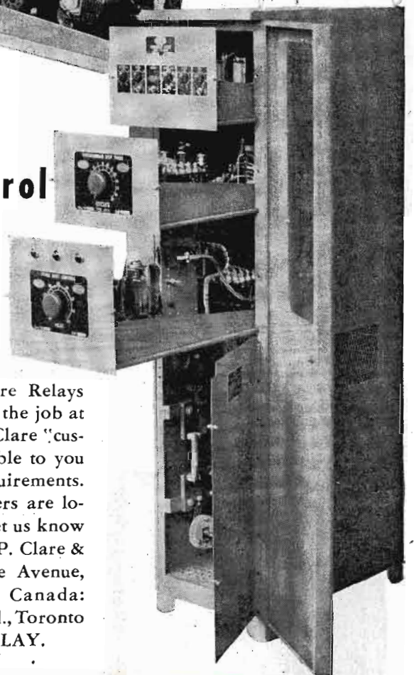
Illustration shows use of Clare Relays in Raytheon Synchronous Control Cabinet
