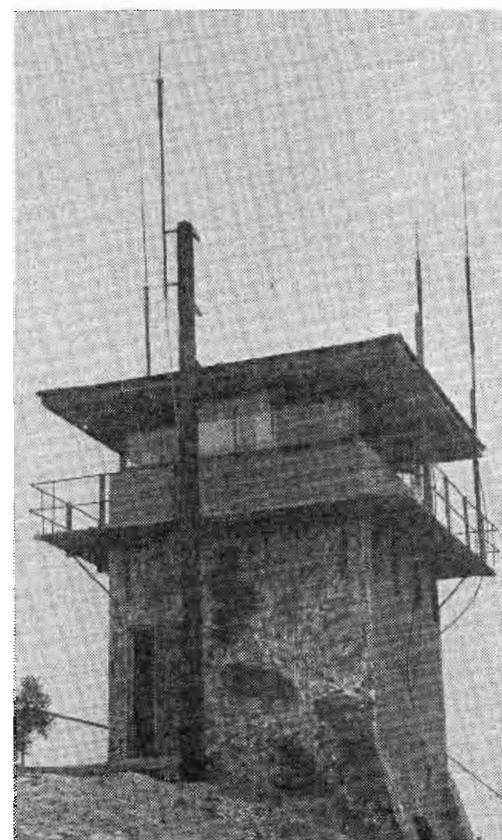
• Below, two sets of relay antennae used by the California Highway Patrol and Ventura County at Ventura, California. The longer antenna picks up signals from cars at 39.78 mc from 30-watt transmitters. The short antenna beams signal at 118.5 mc to the main station in the valley below, approximately forty miles away.
