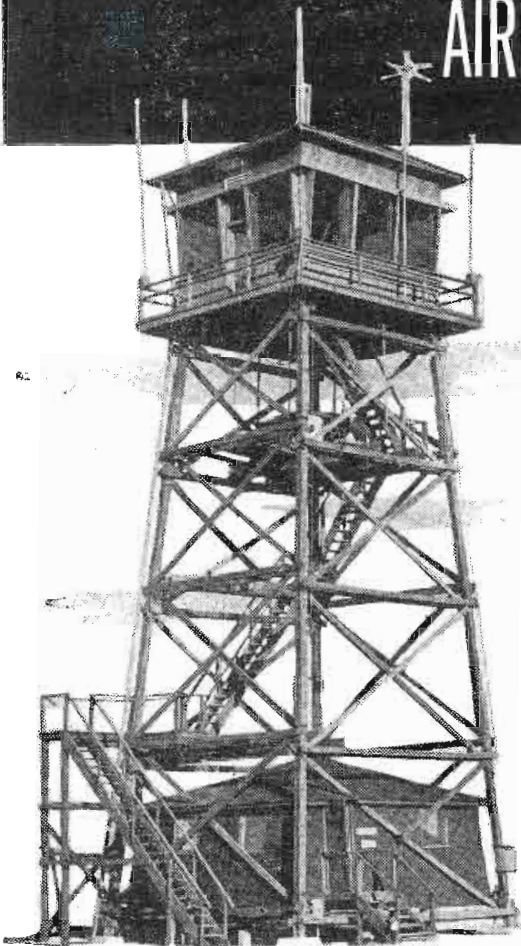
Signal Corps Photo Airdrome Traffic Control Tower some- where along the lines of the Army Air Forces. Operated by the Army Airways Communications System Wing. Main- tains two-way communication between airfield and aircraft.
