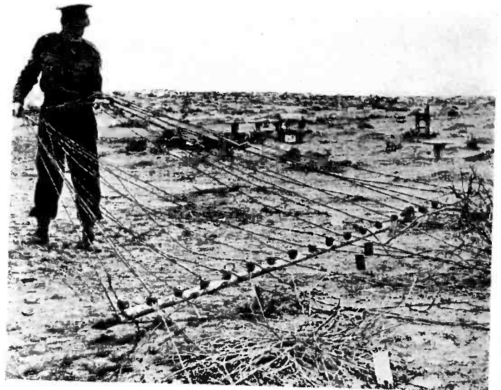
Figures 4 (right) and 5 (bottom) British signal man in Tripolitania testing ground cable junction (Figure 4). A communications switch well, in the Western desert of Africa, protected by a trench (Figure 5).
