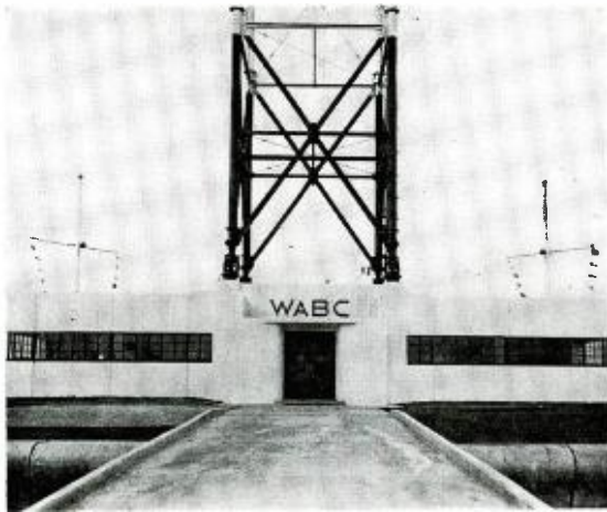
Approach to building. At right and left are the flagpoles, which also serve as emergency antenna. Although the base of the master antenna appears to be secured to the building, it is in reality held to huge pillars that run through the building.
