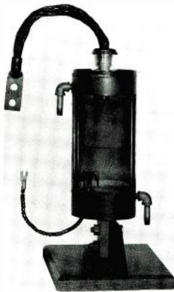
Figure 4 Ignitron for welding control.
