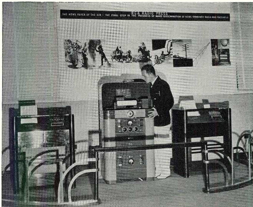
Showing the facsimile receivers and transmitter (center) at the RCA Exhibit, New York World's Fair.
