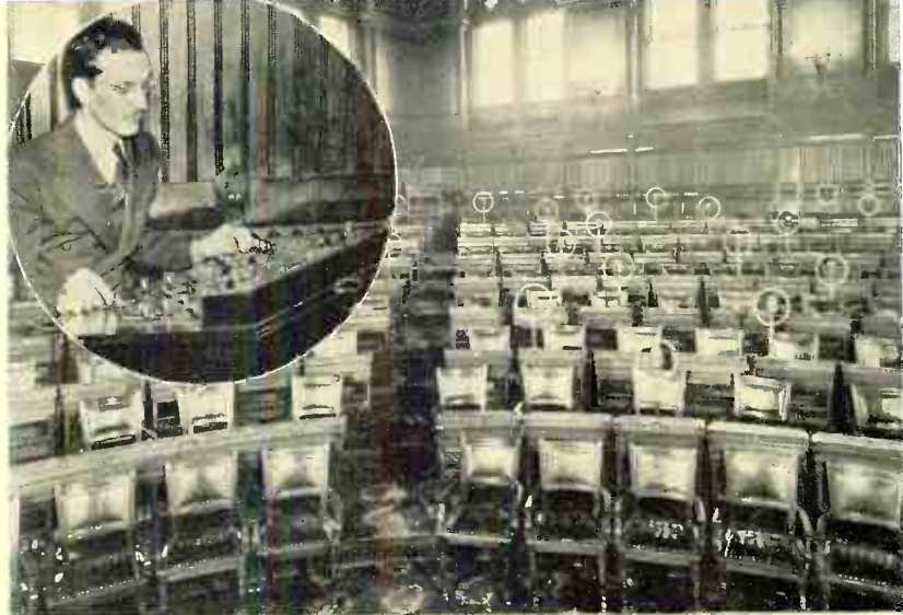
Fig. 9. (Right) The sound system in the Connecticut State Capitol successfully overcomes the former serious problem of dead spots and reverberation. Inset shows the control panel which brings individual microphones into action as required.
