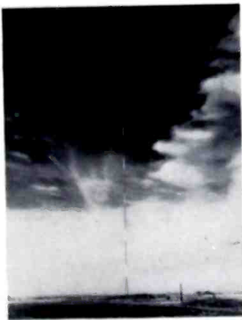
The 445-foot Lingo tubular steel radiator at WIBW, Topeka, Kan.
