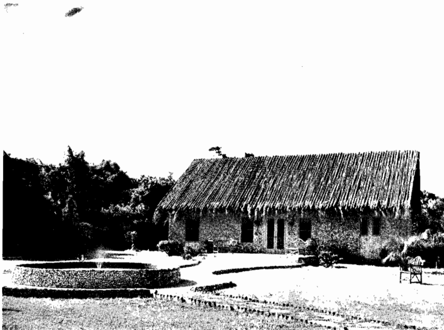
This quaint old "tabby" house, built of oyster shells and covered with logs and Spanish moss, houses the transmitter of WFOY.
