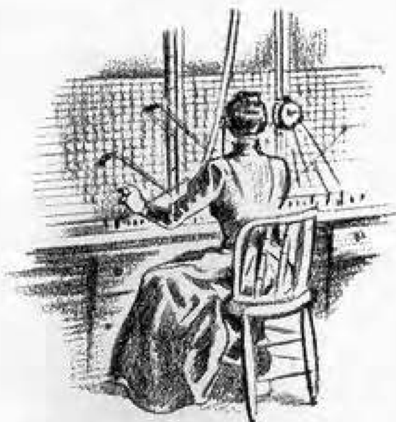
A Western Electric switch- board of the early '80's.
