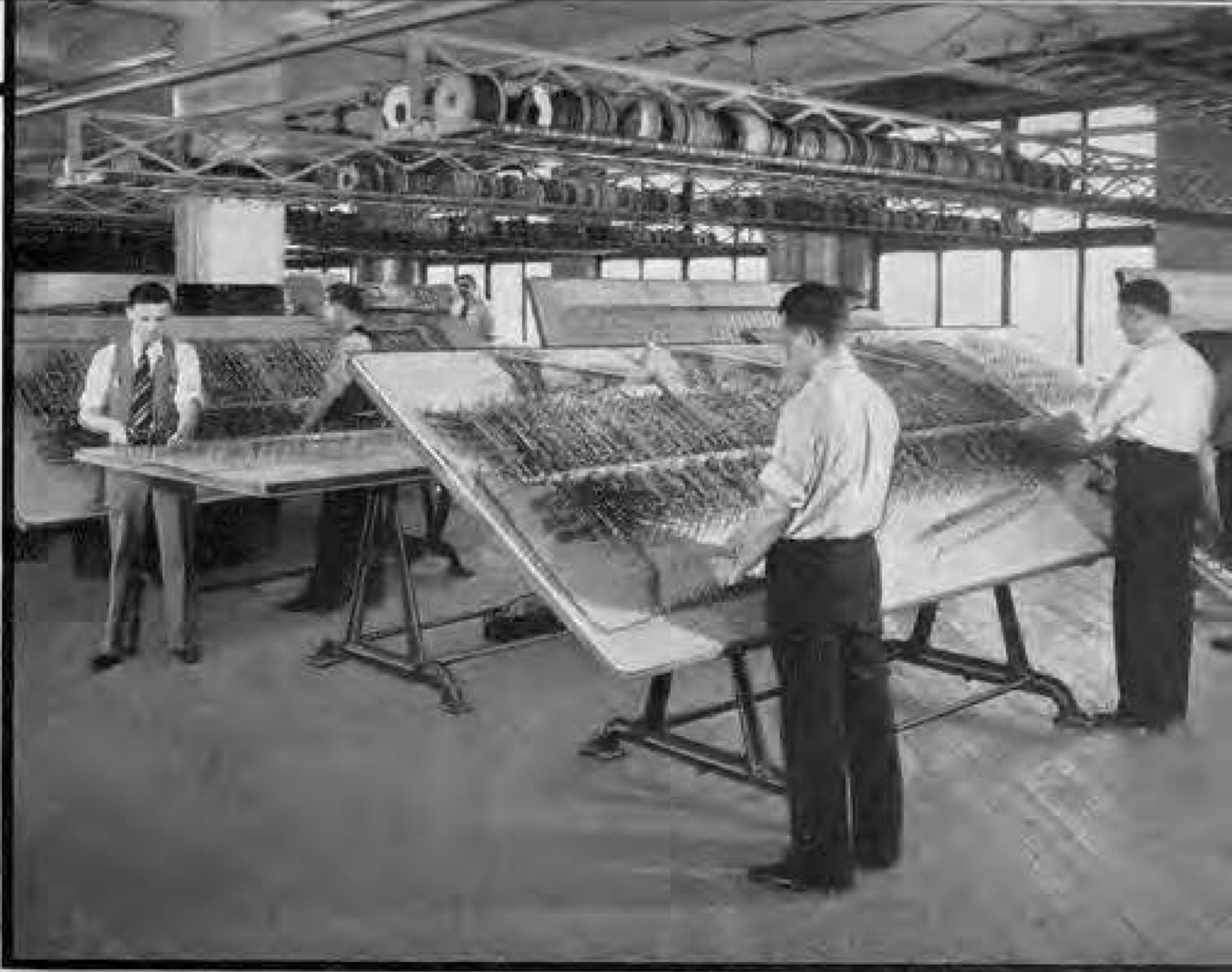
The intricacies of forming dial central office cable.
