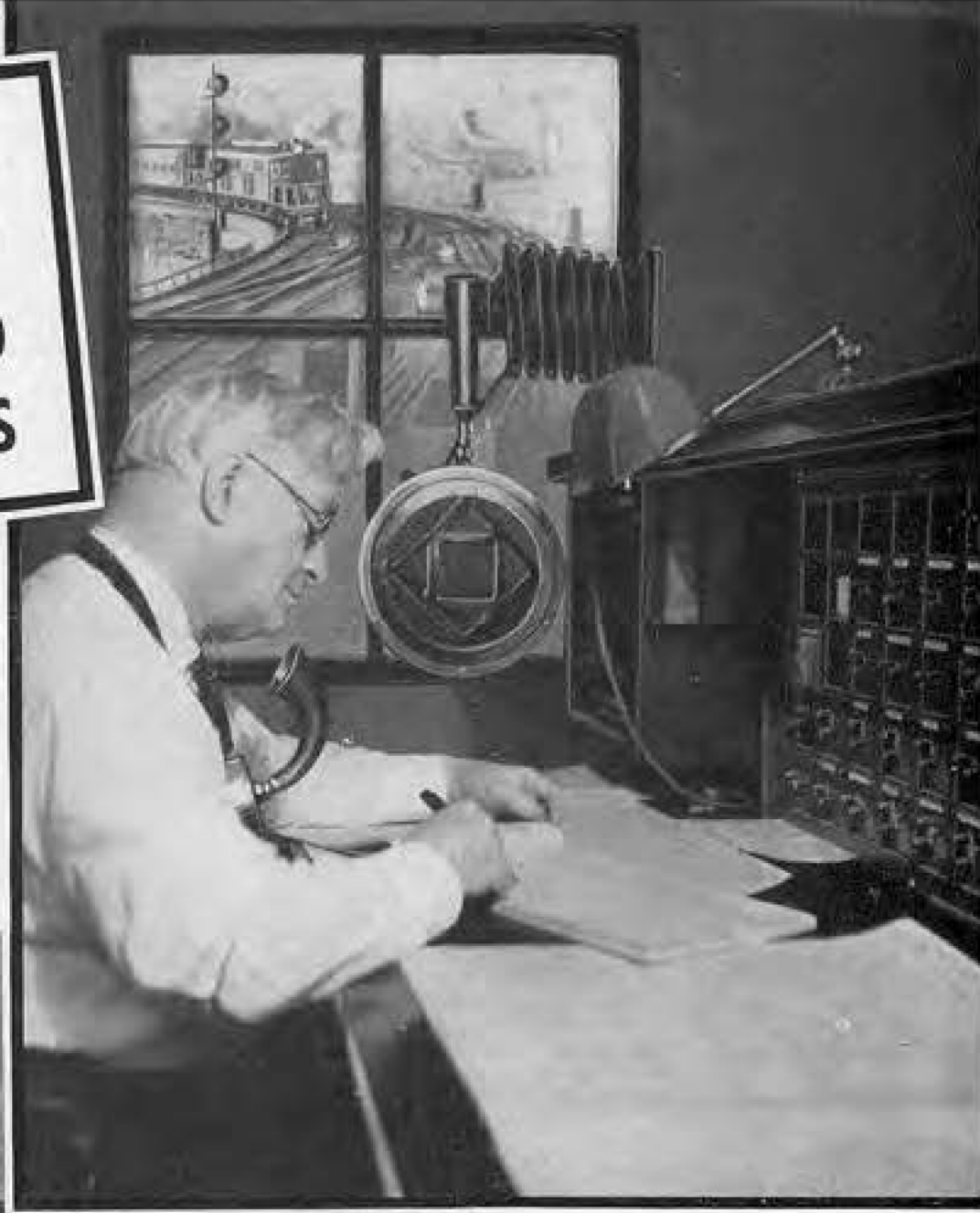
Western Electric telephone equipment and the Teletype for the dispatching of trains.
