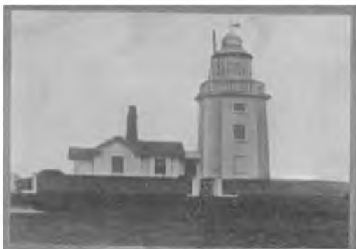
Trinity House Beacon Stations use Marconi Valves.
