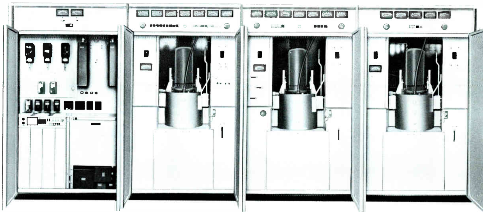
Transmitter control cabinet at left houses exciter/modulator unit and twin, solid-state intermediate power amplifiers.
