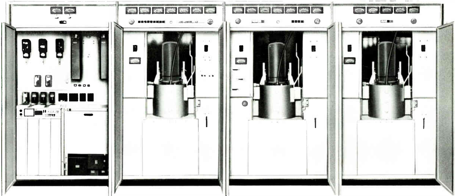
Transmitter control cabinet at left houses exciter/modulator unit and twin, solid-state intermediate power amplifiers.
