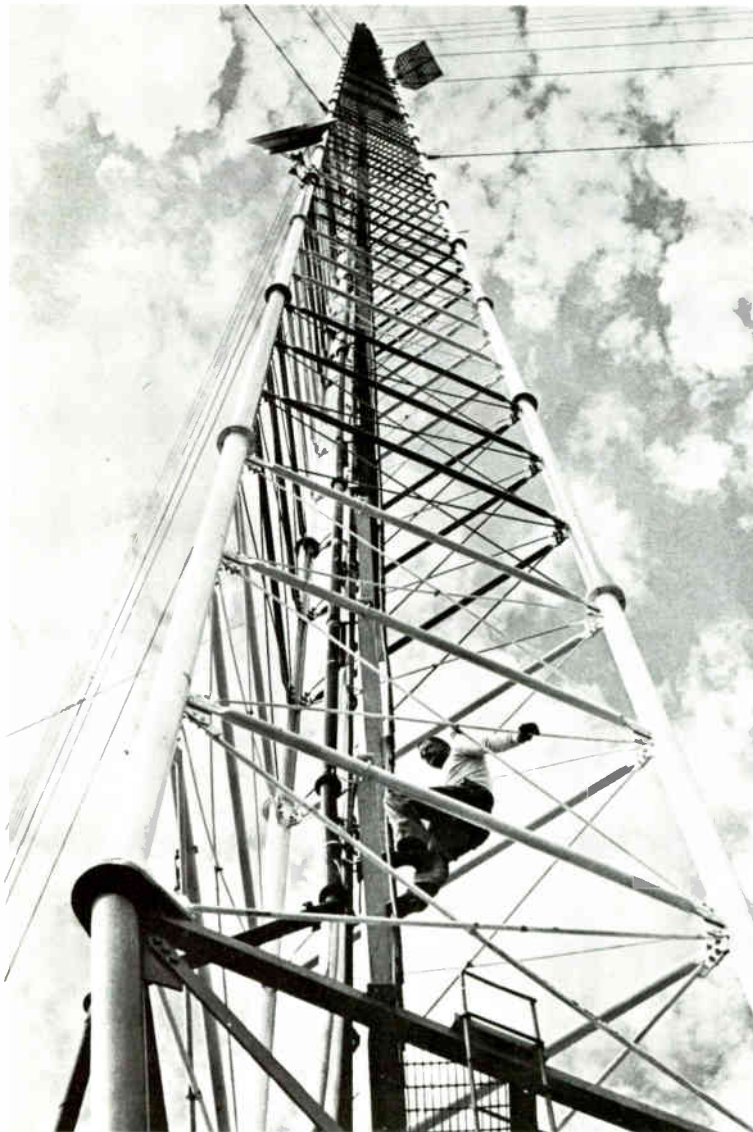
Guyed television towers can achieve great height at less cost than self-supporting structures where land value is not a determining factor. Towers are triangular and are available with either fixed or pivoted base.
