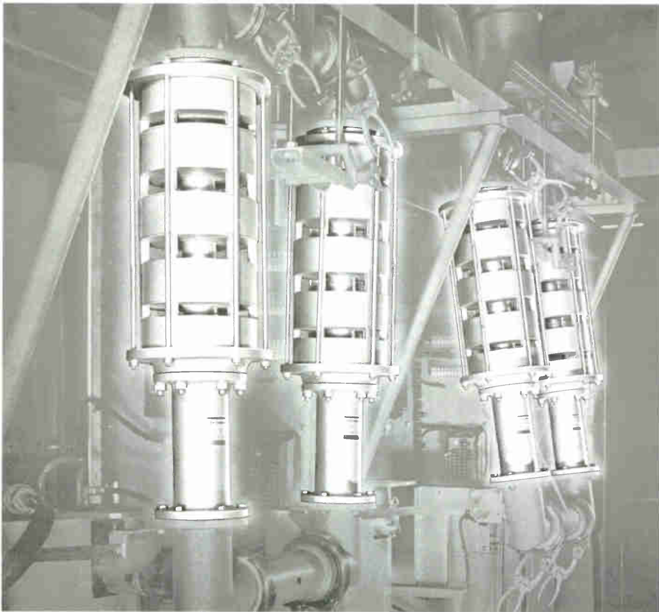
Four harmonic filters in use in an RCA transmitter.
