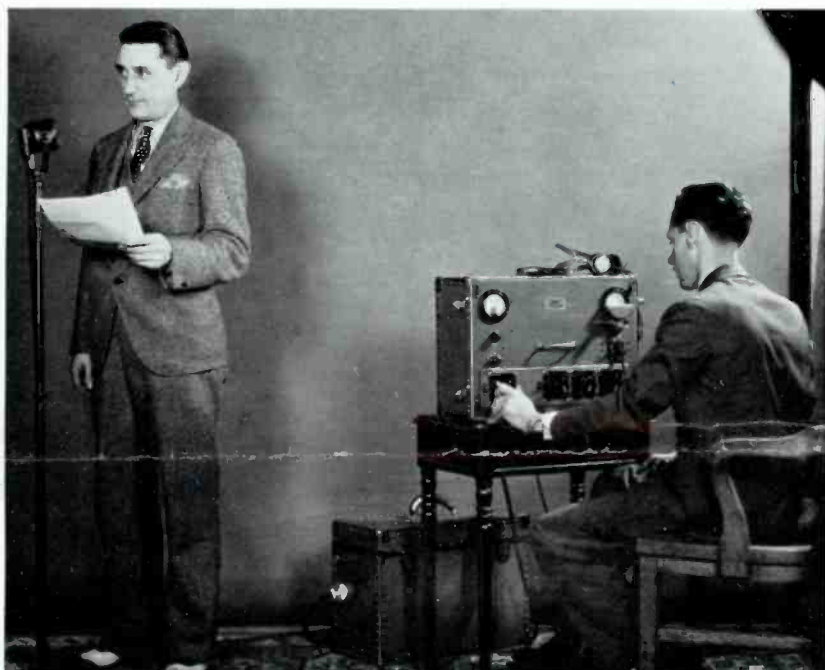
THE NEW —The modern RCA Victor Type OP-4 equipment. A complete portable speech input system, using the Inductor Microphone for high quality outside pickups.
