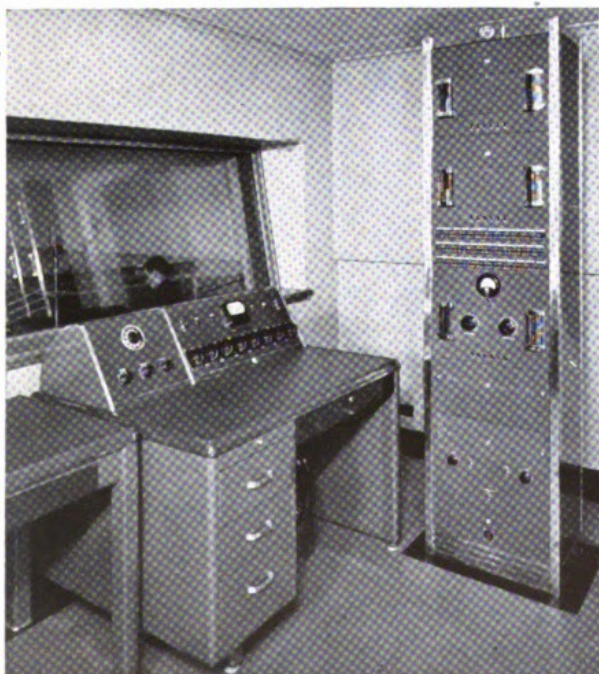
A Studio Control Console and Rack built for WFBR, Baltimore, Md.
