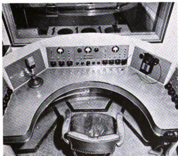
Control Console at W/WNC.
