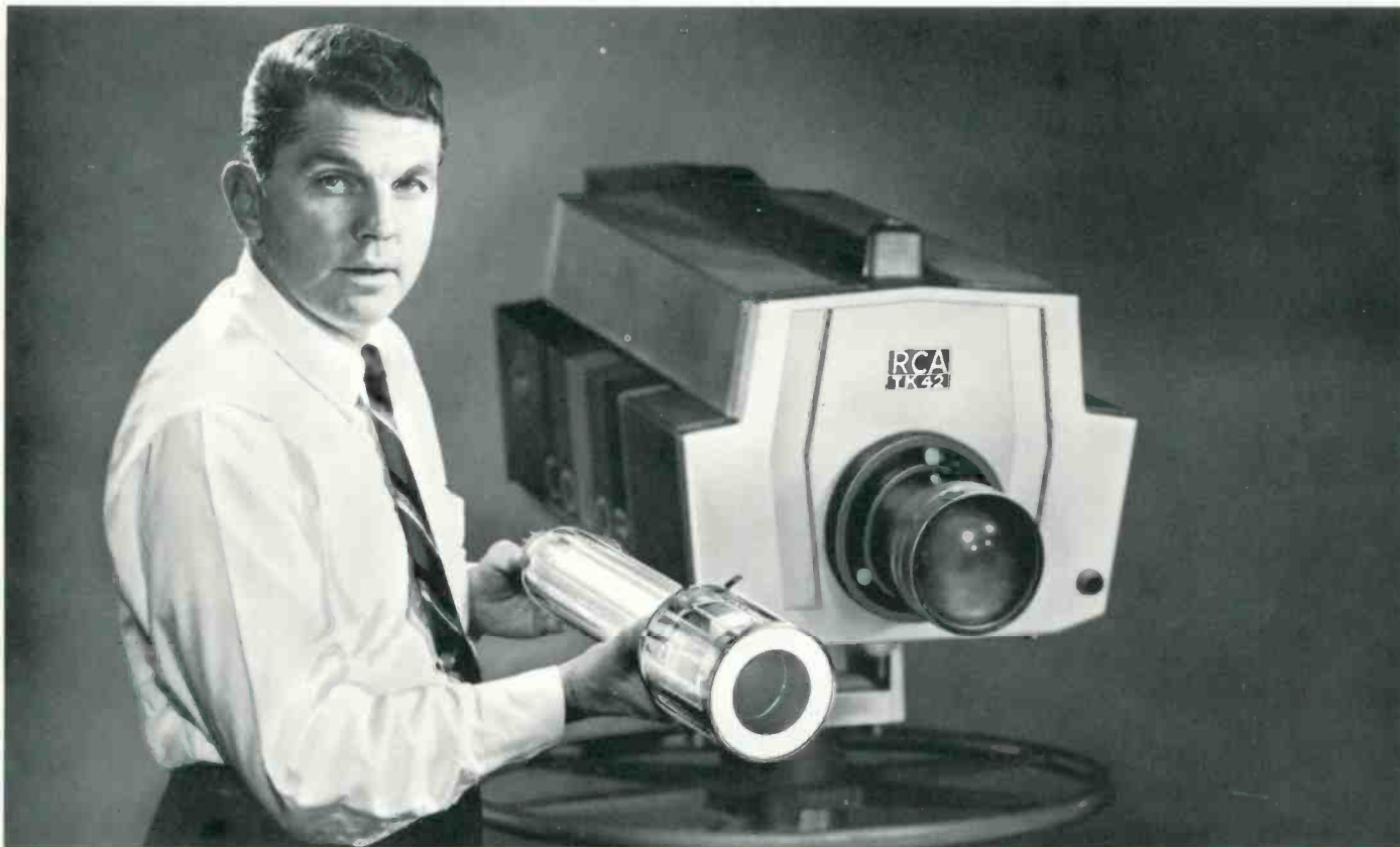
SEPARATE LUMINANCE CHANNEL lends "snap" to the color pictures derived from RCA's TK-42 Transistorized Live Color Camera. Shown above is a 4½-inch Image Orthicon Tube that provides monochrome picture quality equivalent to that of the finest black-and-white cameras.
