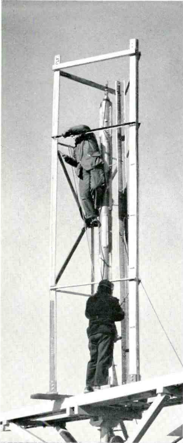
FIG. 12. Pattern test set-up for UHF custom antenna mounted within a tower.
