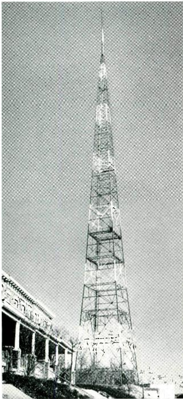
FIG. 3. Self-supporting tower of WBAL-TV, Baltimore, Md. Note the small amount of land area involved and the proximity of tower to residential area.
