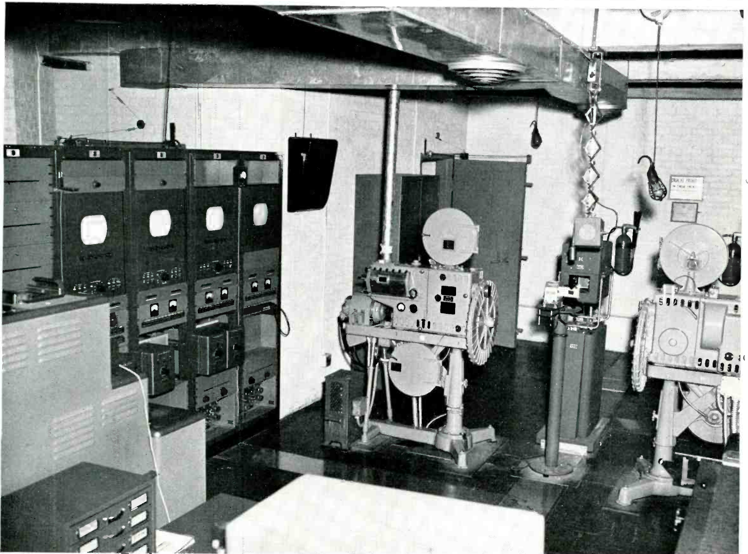
FIG. 25 (below). View of one end of the Projection Room; the two 35mm projectors and the projection room monitoring racks at left with the TM-1A picture monitors mounted at top.
