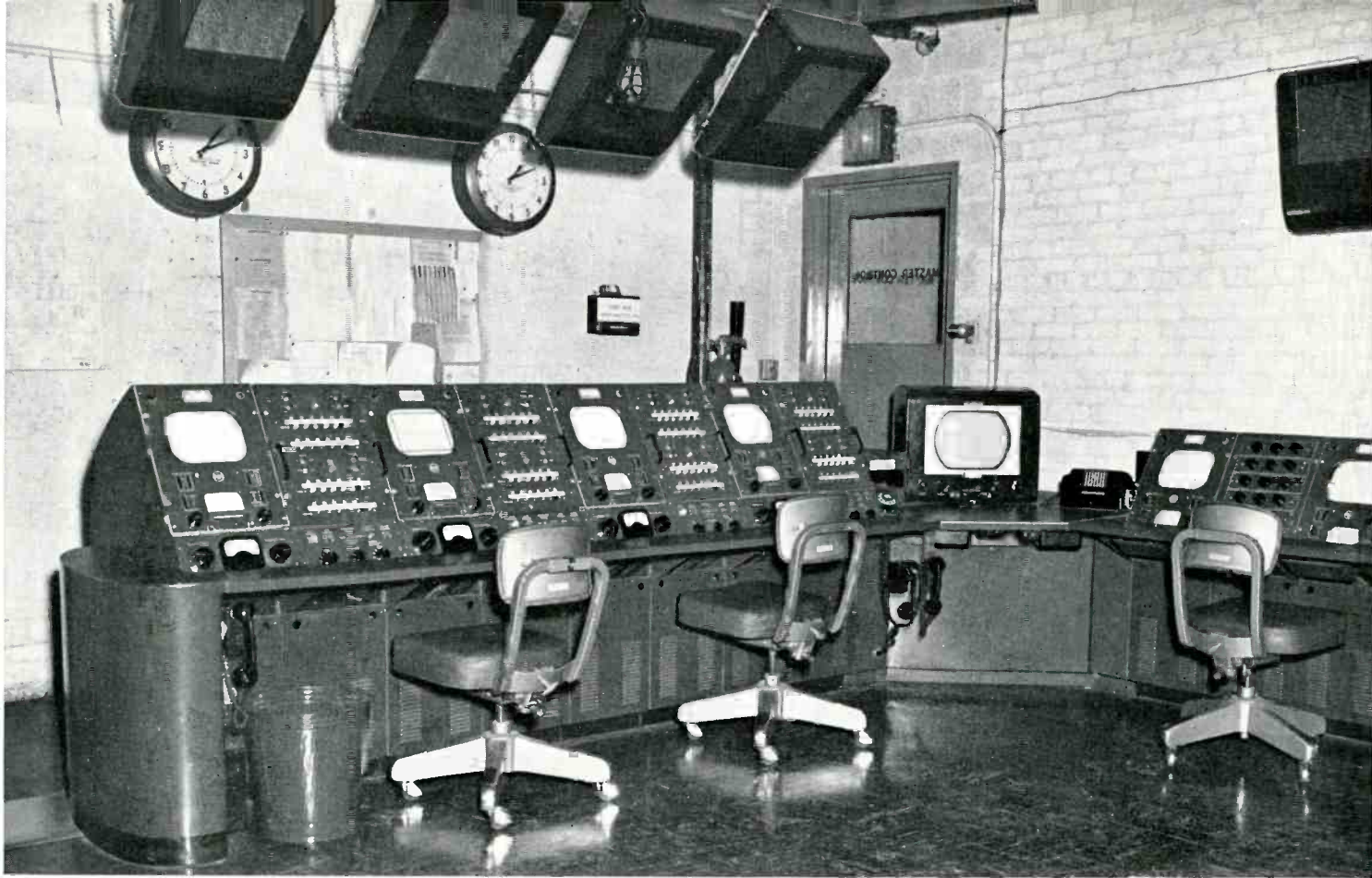
FIG. 31. Front view of the WOR-TV Master Control Switching Console which consists of facilities for switching six incoming circuits to four outgoing channels.
