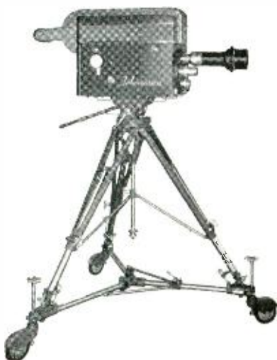
Dolly Fitted to Camera Tripod, TD-11A
