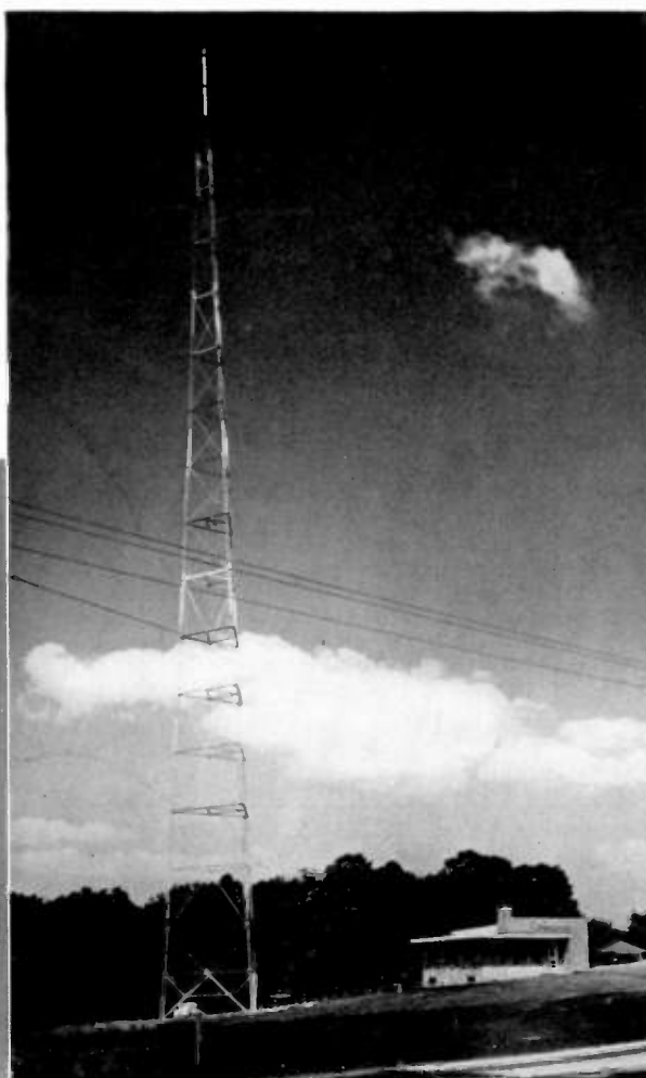
Tower and two-section Pylon at WSB 3 -FM, York, Pa.
