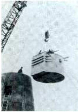
Inset: Positioner Being Lifted Into Position
