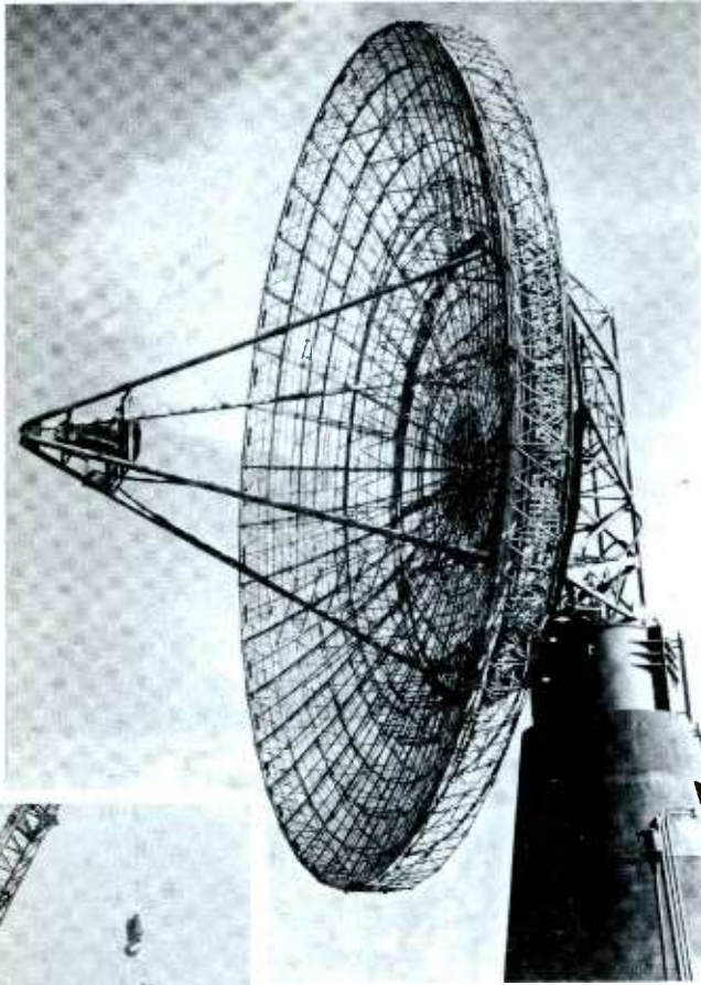
Complete Installation of Rotatable 60 Foot Tropospheric Antenna and Positioner
