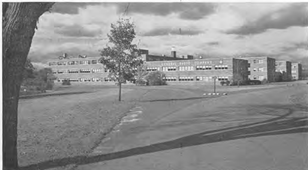
View of General Radio plant in West Concord, Massachusetts.
