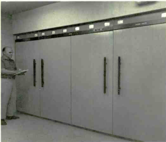
KDAY, LOS ANGELES —The first station to employ Gates VP-50 Vapor Cooled 50,000 watt AM transmitter.
