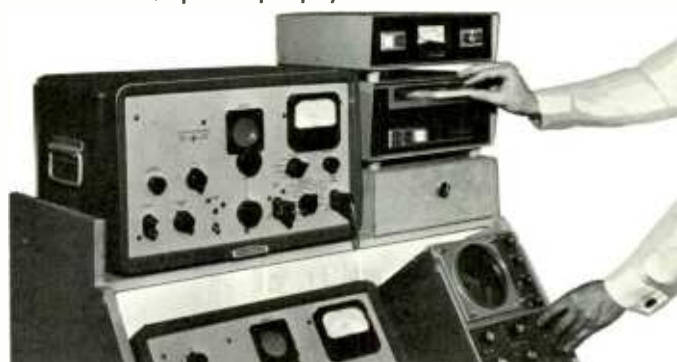
Each cartridge is tested for recovery level of recorded tone to assure stable levels from cartridge to cartridge.
