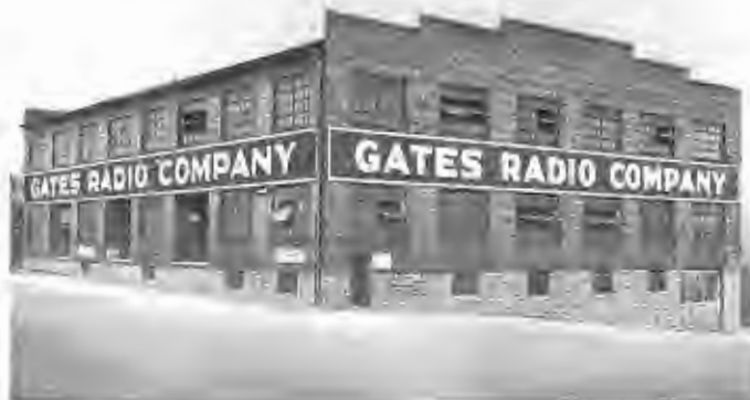
Gates warehouse and regular shipping point. It is one of the most strategically located buildings in Quincy in relation to air, rail and truck shipping.
