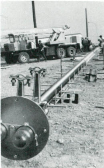
Pole and accessories assembled on ground prior to erection.
