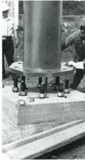
Pole in position to be lowered on plumbing nuts.
