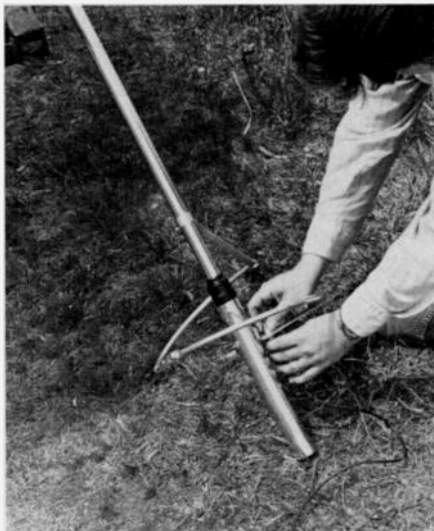
One of the first things you should do before you put up your antenna is insert the coax. It makes things lots easier.
