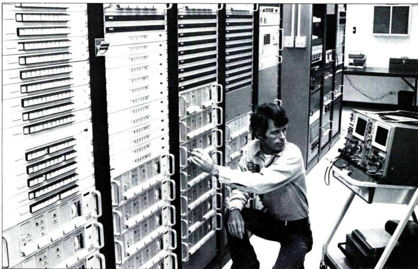
Richard Keith, a technician for UA-Columbia Cablevision, adjusts the output level of an RCA color television modulator at the headend facility in downtown San Antonio.
