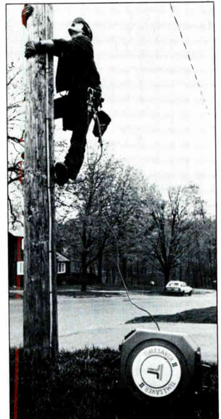
Times Wire & Cable's dispenser-refill system for protecting and installing drop wire.
