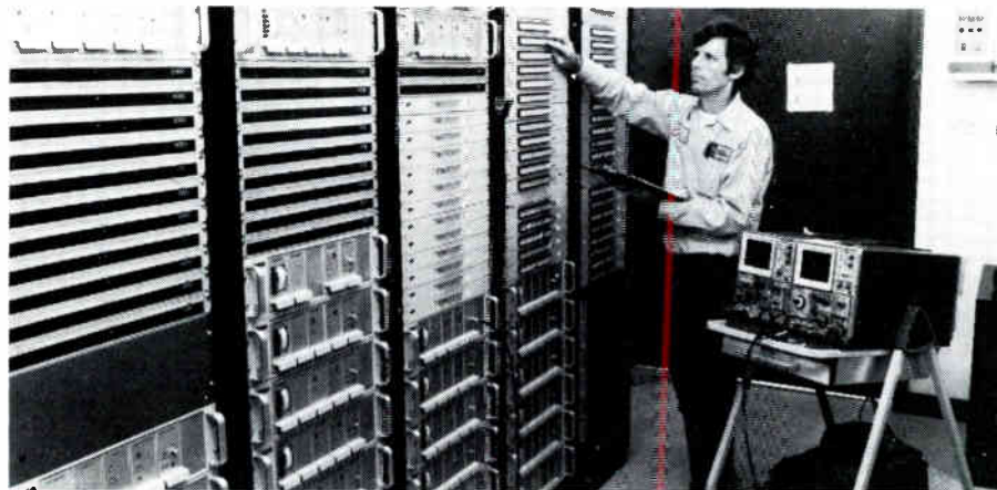
Final adjustments on the UACC headend are made by technician, Richard Keitr. The central-hub headend is situated atop the 21-story NBC building in downtown San Antonio. The 32-channel headend utilizes RCA CTM-10 Modulators and CTD-10 Demodulators.
