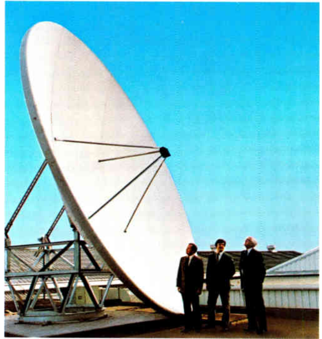
Times officials examine new 7-meter satellite antenna at the company's Wallingford, CT headquarters plant. The TVRO is used for experiments and to test fiber optic satellite downlinks.
