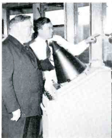
Figure 2. Aboard the Great Lakes steamer "A. H. Ferbert," Capt. Frank Davenport (left) listens while C. E. Moore of Radiomarine Corp. explains operation of new marine radar gear. Indicator unit in foreground has a "daytime" hood over the 12-inch oscilloscope on the face of which the radar image appears.
