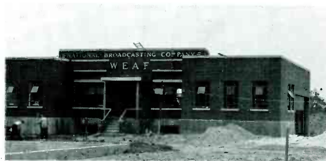
The New WEA F Transmitter Building
