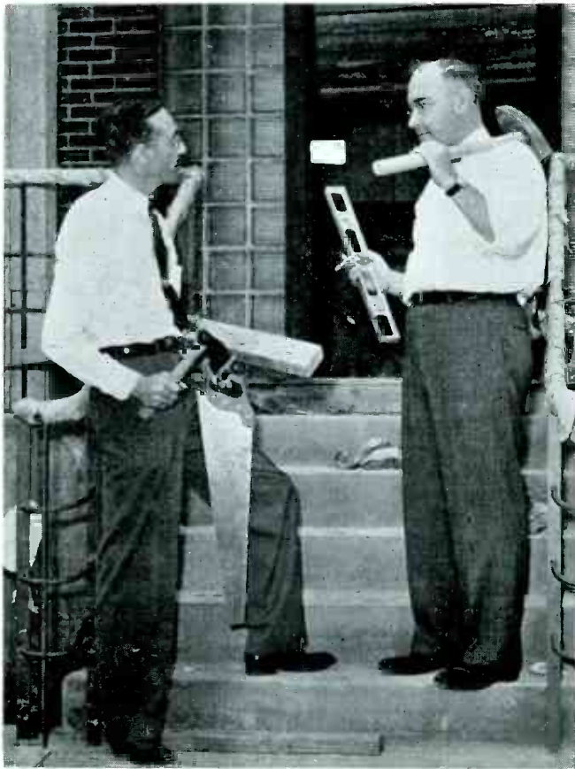
Messrs. Hanson and Guy step outside the new WCAF building to settle a difference of opinion. They compromised by sawing off the foreman's leg, and wrecking the building.
