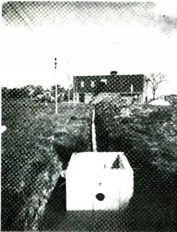
Center manhole to the main tower.
