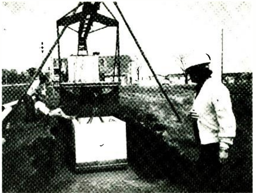
Dave Pierson (right) supervises the placement of the pull box.
