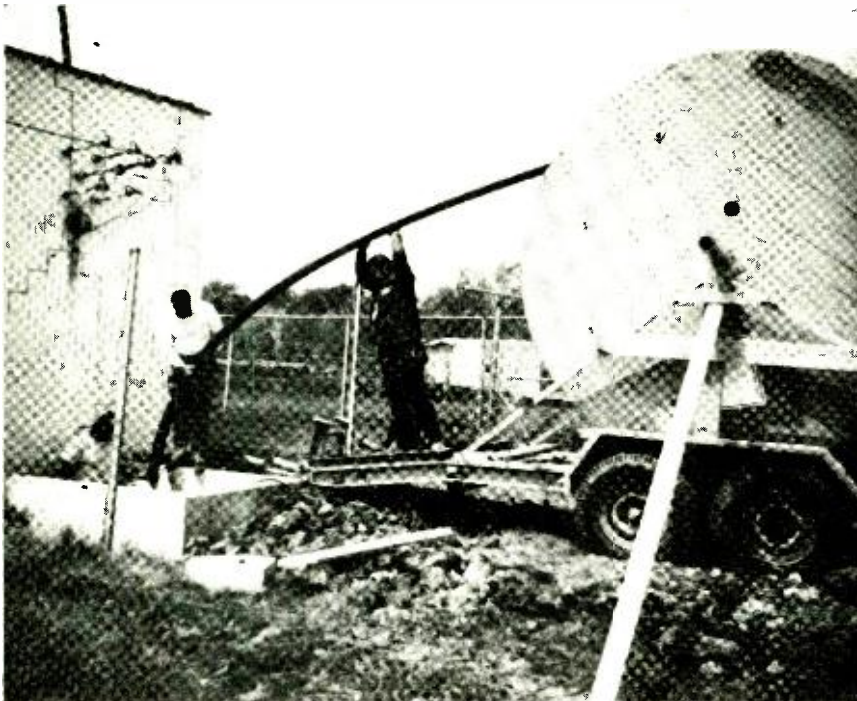
Installing the 4 1/8-inch coaxial cable.
