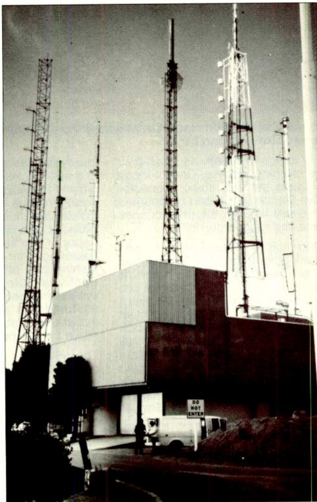
High winds may pose a danger to some towers.
