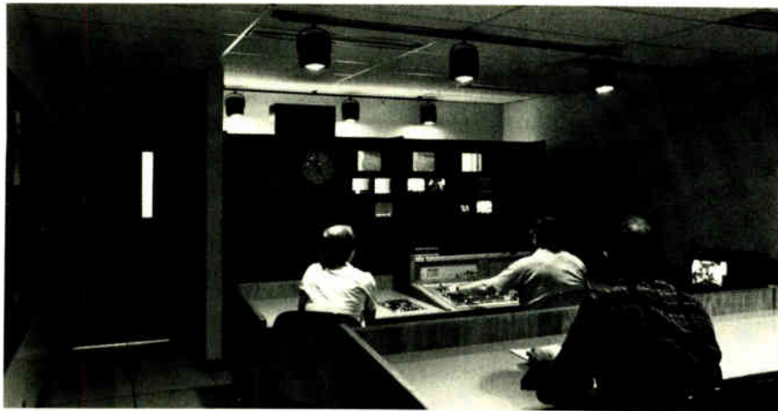
Track lighting in production control keeps light off Sony and Panasonic monitors and focuses it on work areas.
