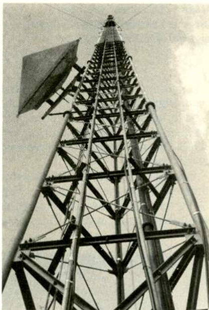
The antenna at KRNE-TV, near Merriman NE, is 1029 feet high.
