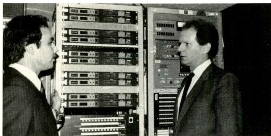
Kevin Dauphinee (right) and equipment planning engineer Achille Raspantini inspect a bank of Lexicon 1300 digital audio delay synchronizers at the network's New York central control.
