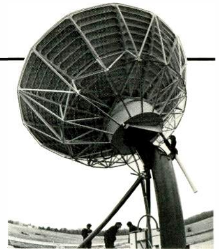
WHAS's nine-meter Harris dish, located near Eastwood, KY, is controlled by a computer that is remotely programmed from the station's facility, 18 miles west in Louisville.
