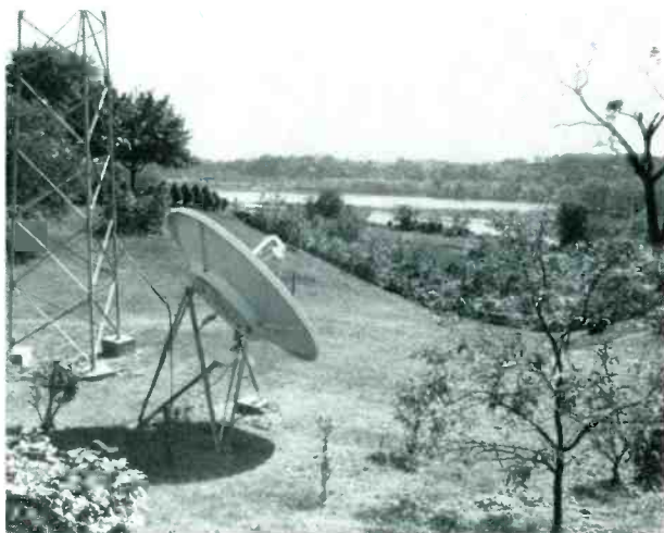
California Microwave dish, at base of tower, picks up Mutual news broadcasts.
