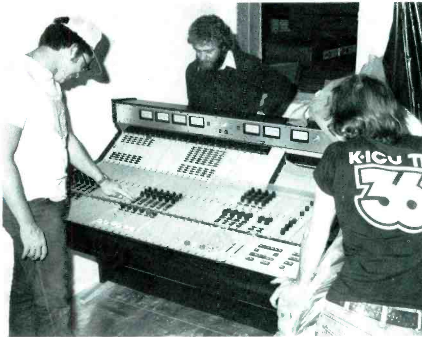
Increasing attention to TV audio is reflected in KICU's installation of an ADM 2400 console.
