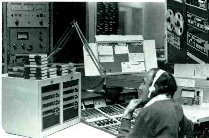
The WJTN-AM control room and master control position with easy visibility to metering. This studio features a McCurdy console, two ITC triple decks, Eventide time delay, two turntables, and five Revox A77s.
