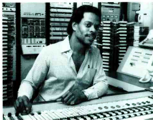
Engineer Michael Beatty operates Pacific Recorders console in master control. In back of him are modified Instacart, jack fields, other rack-mounted units.
