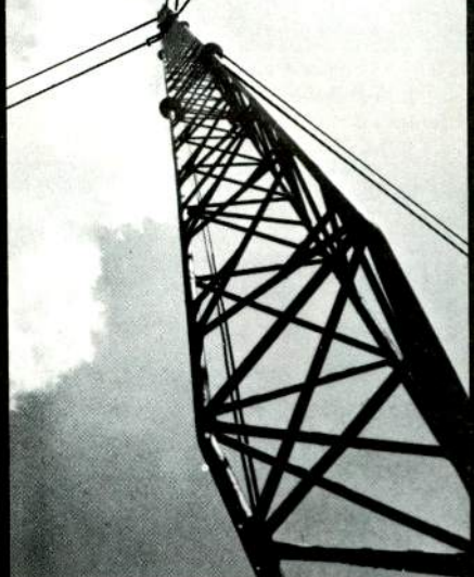
Phillystran® HPTG installed on WORL in Orlando.
