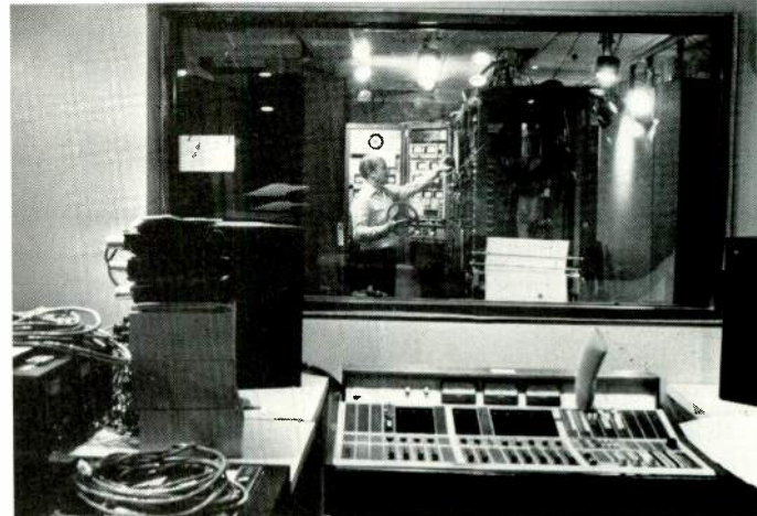
Quality assurance in radio starts with design that allows proper control of operation. In the well laid out studio above, control position and technical area have close eye contact for instant communication
