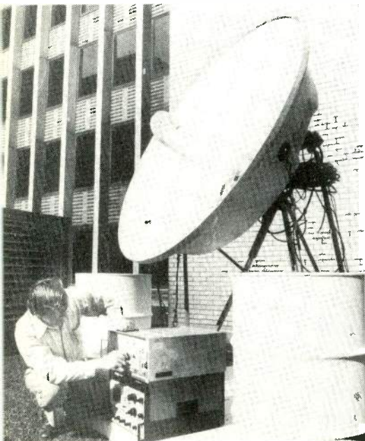
Six-foot satellite antenna on office roof.
