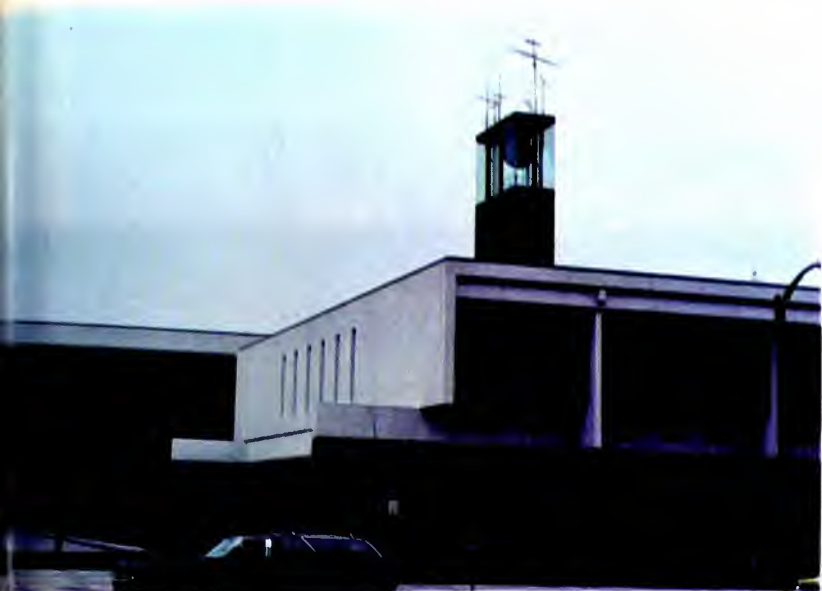
Exterior of new WGR-TV studio-administrative building in downtown Buffalo has brick facade on first floor, tinted windows above. Glass-enclosed tower holds microwave antenna for air link to transmitter.
