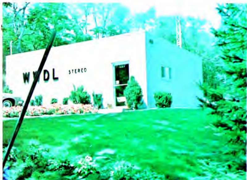
WWDL's old building, with 800 square feet of floor space, before the expansion program that incorporated it into the new building, shown in lower photo on opposite page, extends across one end of the old, with a new entrance at far right.
