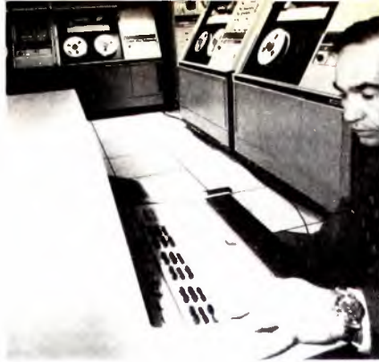
VTR room has four AVR-1 and two VR-1000 Ampex videotape recorders. Ampex RA4000 editing console is in foreground.
