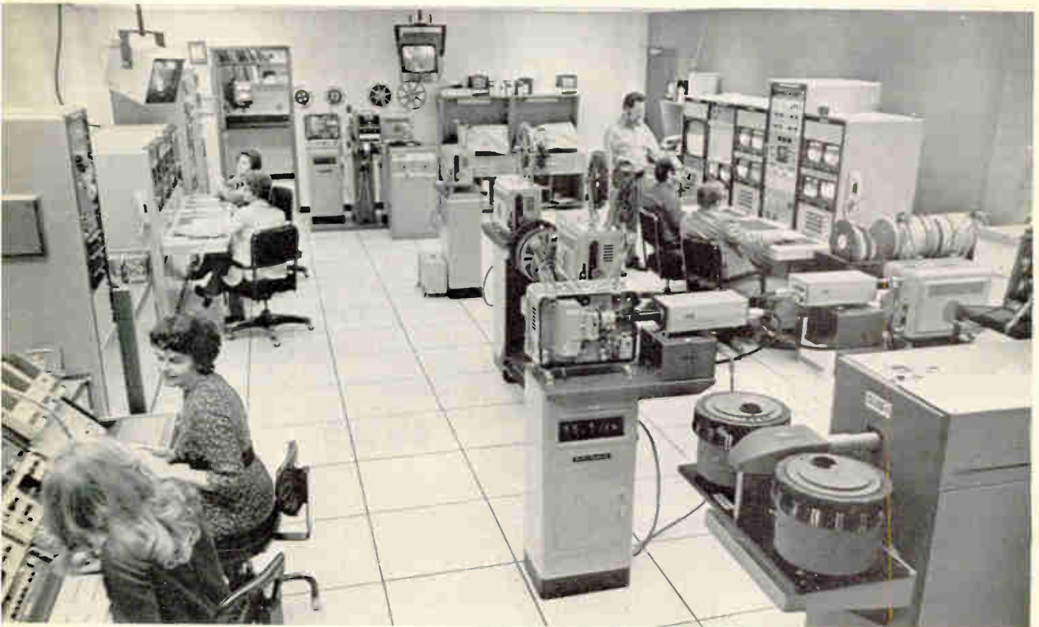
Overall production area view of the Master Control Room. Master Boards to the right, LPC across the room on the left, and the production consoles in lower left.
