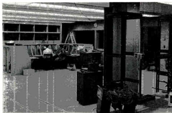
Note use of computer floor eliminating wiring trenches. Photo taken during construction phase.
