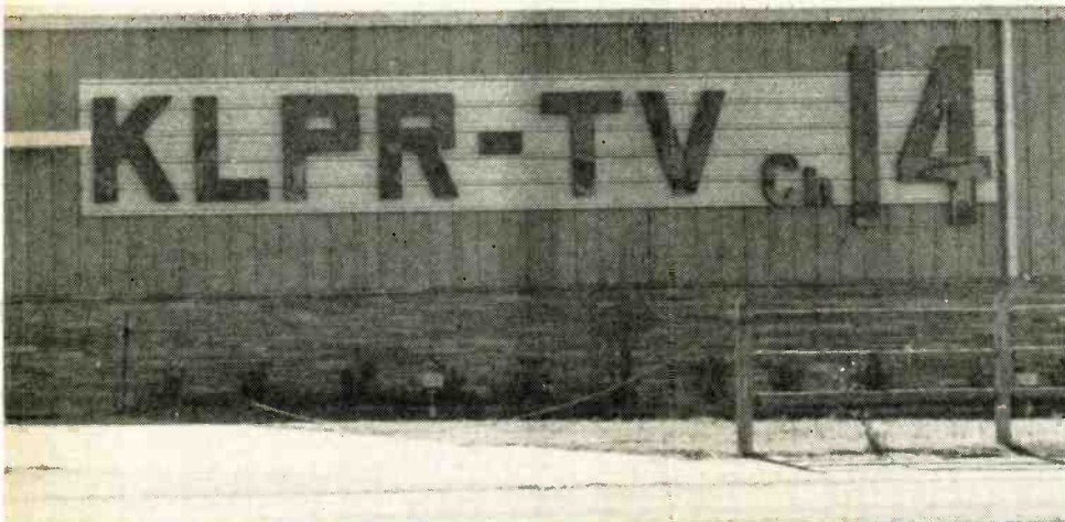
Studio and transmitter building is modest, but serves the purpose.
