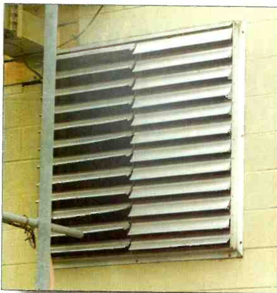
Unprotected louvers such as these are at risk of freezing shut in icy conditions. Installing a protective shroud can ensure they will work properly regardless of the weather.
