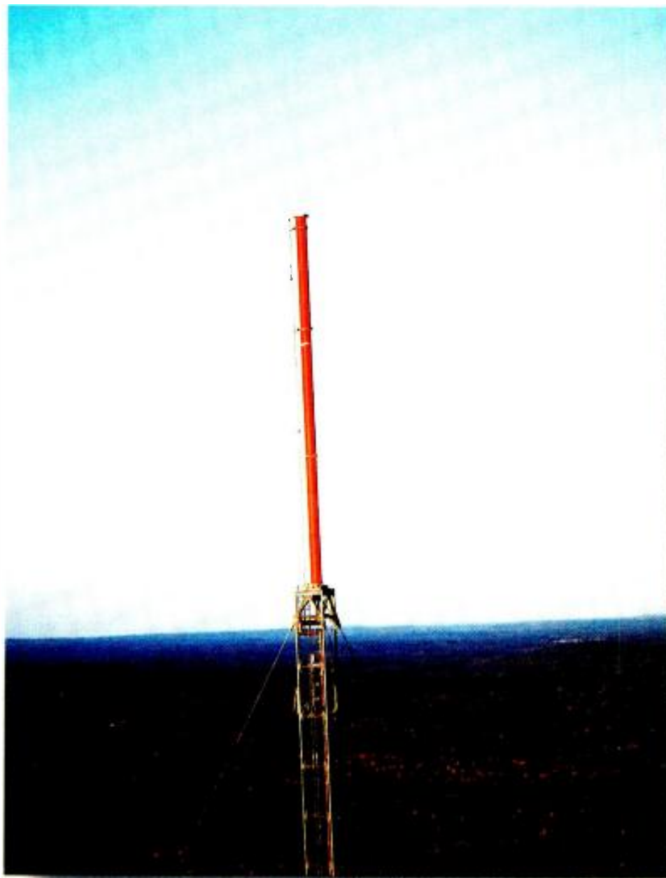
An optimum installation for stations would be a top-mounted omnidirectional antenna. Shown here is an Andrew UHF TRASAR at WPME-TV.
