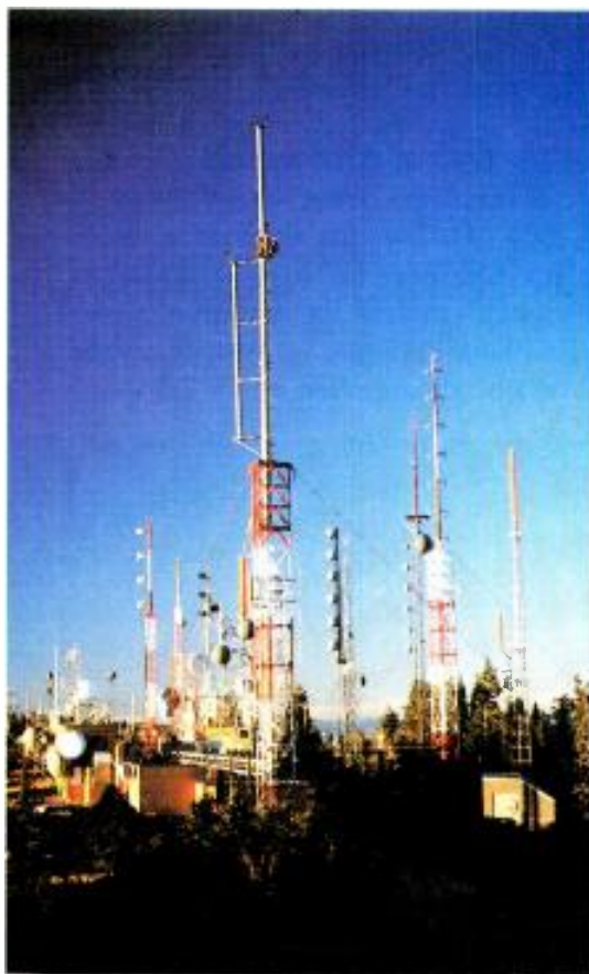
A stacked antenna solution is used by stations' KRQE, Channel 13 (top) and KASY-TV, Channel 50 (side). Both antennas are from Andrew. Note the two riggers working at the base of the top-mounted antenna.
