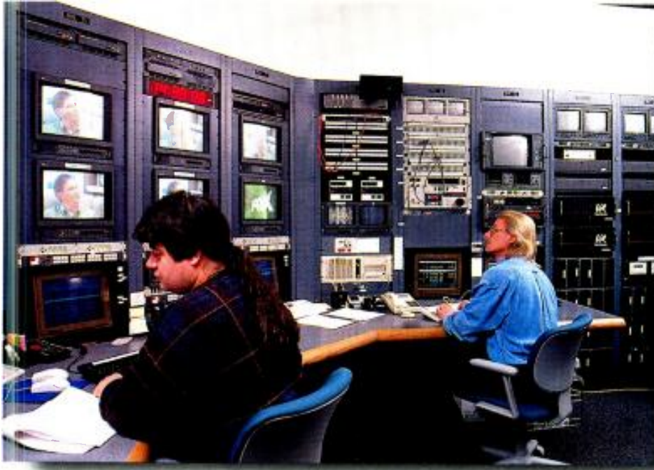
Digital pay-per-view control room for TCI's Head-end In The Sky (HITS) service. At present, the room runs 27 channels, but is capable of handling 36 channels.
