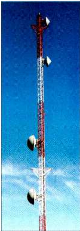
Towers used for a variety of communications purposes are subject to federal obstruction marking regulations, which include rules for paint and lighting. (Photo courtesy of Bob Mosher, CEE, consulting engineer.)
