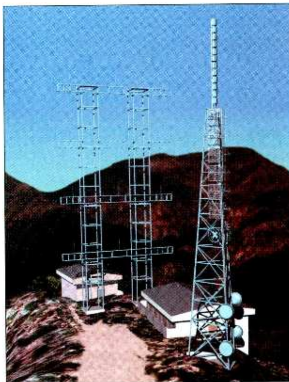
Directional antennas can be used in mountaintop locations, such as this, to direct signals toward population centers and away from sparsely populated areas. (Artist's rendering courtesy of Natural Marketing/Lodestar Towers California, Los Angeles.)
